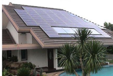
Solar Roof: 5 kW.
