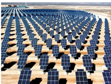
Solar Power Plant: 14 MW.
